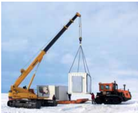
The SENNEBOGEN 643 loading residential containers onto a sledge.
