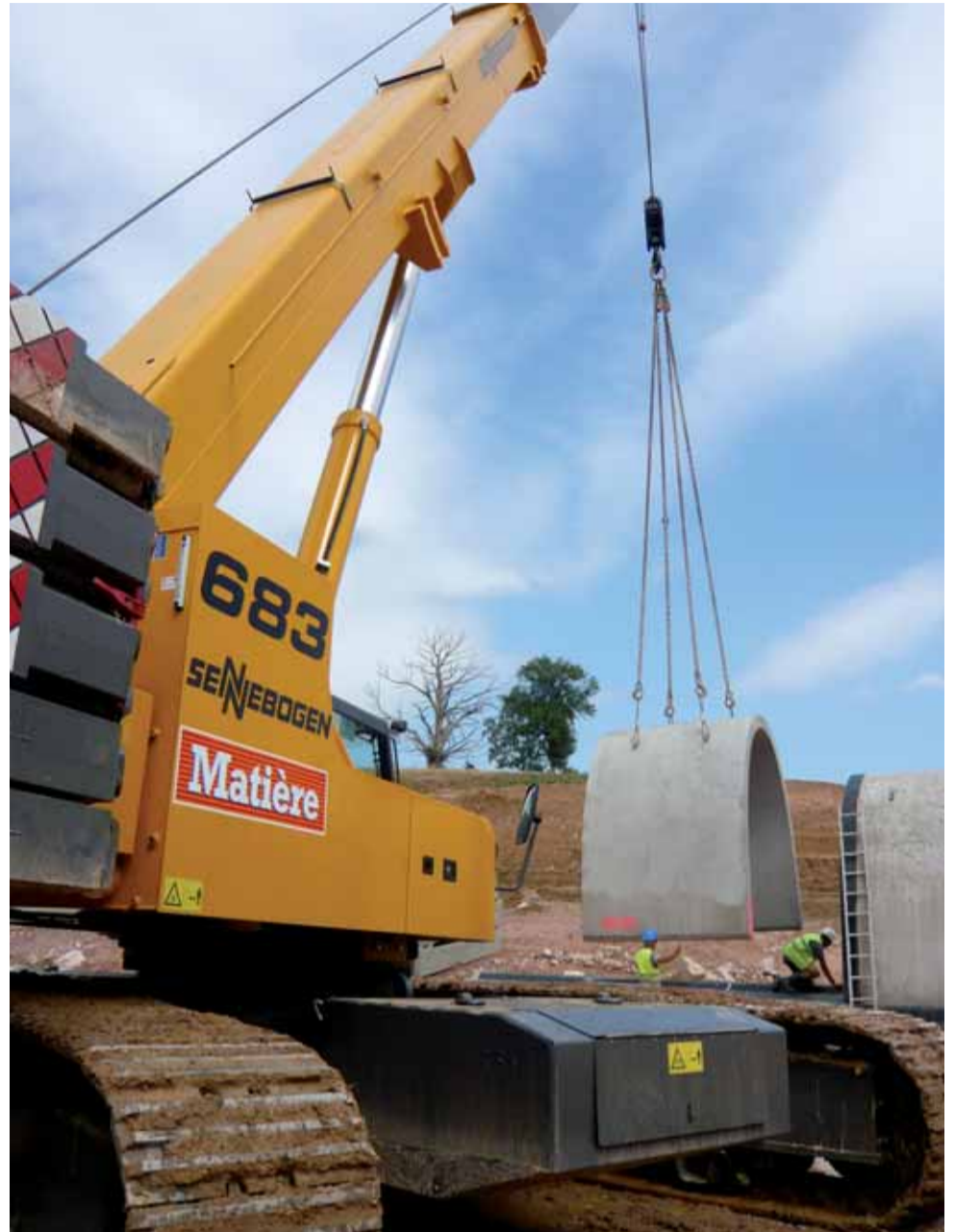
Perfect for assembling the prefabricated concrete parts, weighing up to 25 t. The SENNEBOGEN 683 is ideal for safely lifting, transporting and positioning under load.
