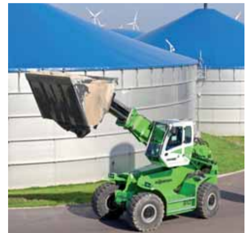
Around 450 t of substrates are distributed to the 16 feeders daily using the SENNEBOGEN 310 and 305.
