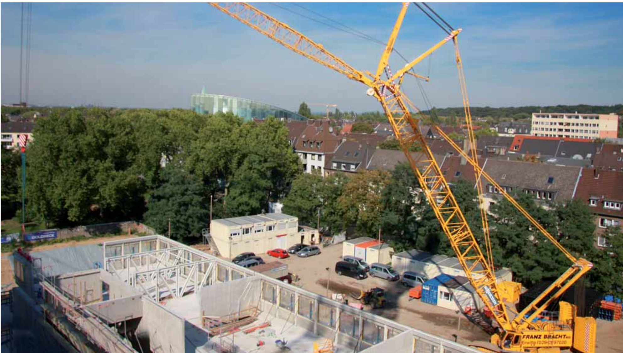
The new SENNEBOGEN 7700 with 300 t lifting capacity into use at the building site for the new Central Vocational College in Duisburg. The 29.9 m main boom and 41.1 m luffing jib creates the necessary large working radius of up to 60 m.
