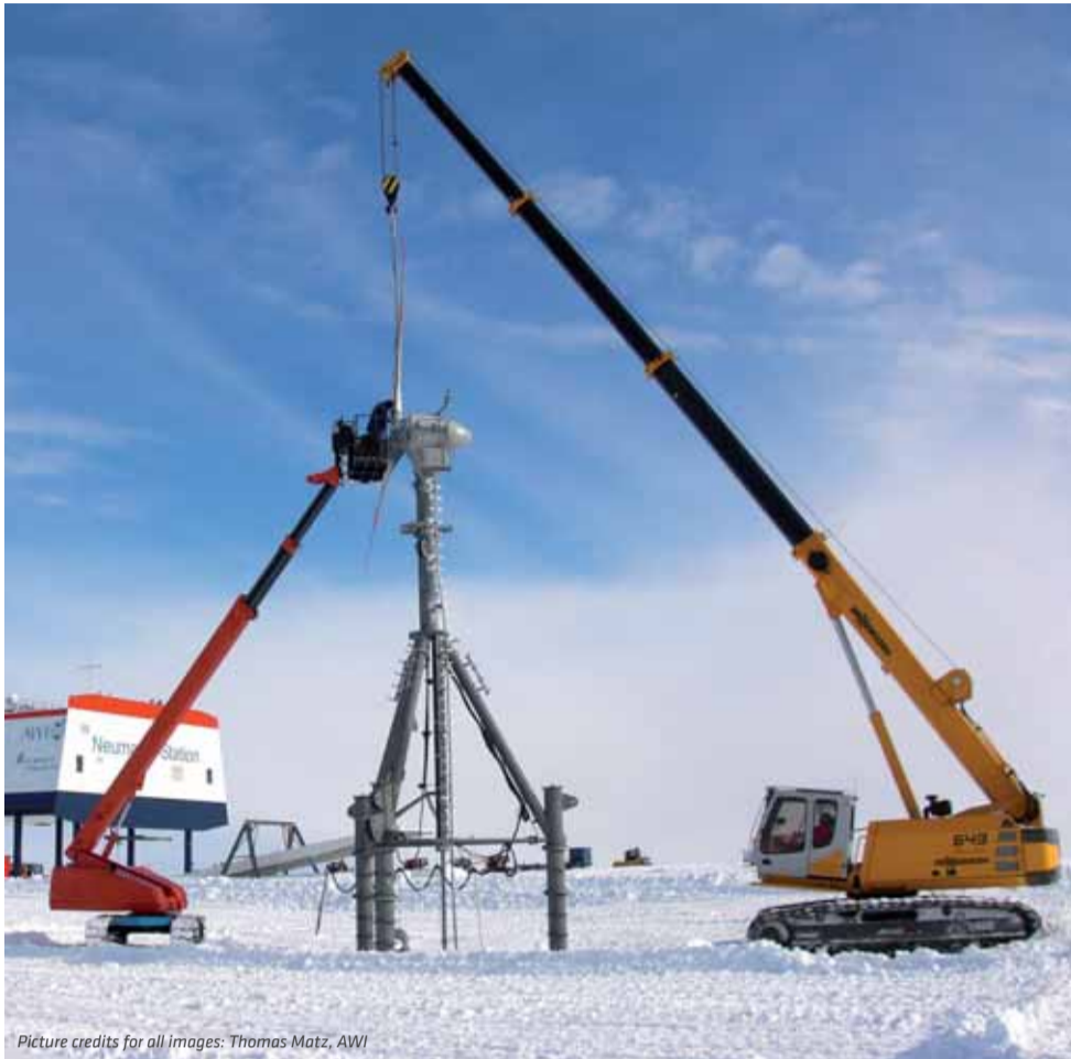
The SENNEBOGEN 643 telescopic crawler crane during the construction of a 30 kilowatt wind power plant.
